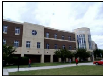
Health Sciences II Building, Main Campus
