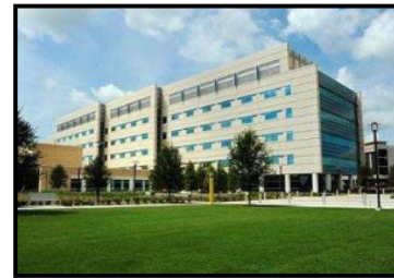
Burnett Biomedical Sciences Building, Health Science Campus
