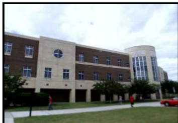
Health Sciences II Building, Main Campus
