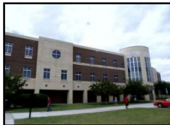
Health Sciences II Building, Main Campus
