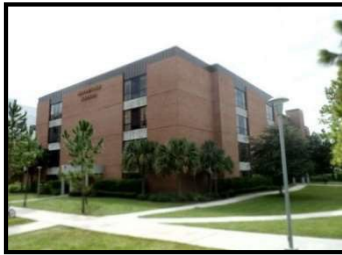
Biomedical Sciences Building, Main Campus
