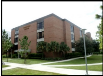
Biomedical Sciences Building, Main Campus
