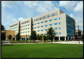
Burnett Biomedical Sciences Building, Health Sciences Campus
