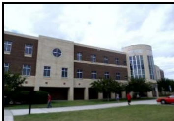
Health Sciences II Building, Main Campus
